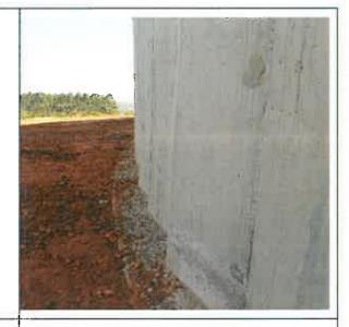
**Picture 2:** jagged edges of reservoir as a result of poor workmanship
